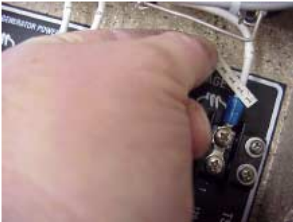
Check the wire markers on terminal strip TS-0 locations: 1, 6, 7, 12, 13 & 15. Re-tag the wire locations if necessary.
